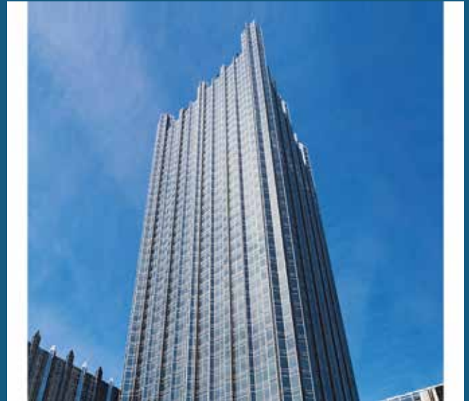
One PPG Place is glazed with 19,750 pieces of Solarban® 550 glass. (Courtesy of Vitro Architectural Glass)
